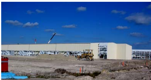
New T-hangars at Page Field near completion.
