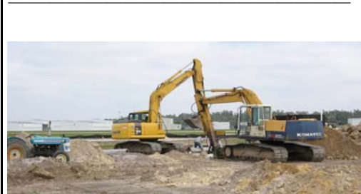
Construction at Delta 2
