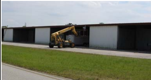
New doors being installed on the Bravo T-hangars
