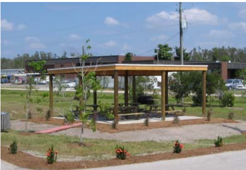
Picnic shelter at the Foxtrot T-hangar complex
