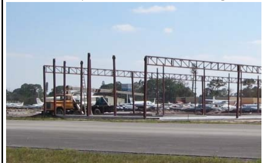
Steel going up at the new T-hangars
