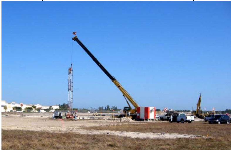
Runway 5 glide-slope equipment being relocated at Page Field recently
