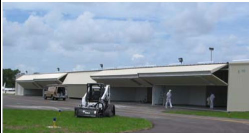
Finishing touches on the Alpha T-hangars
