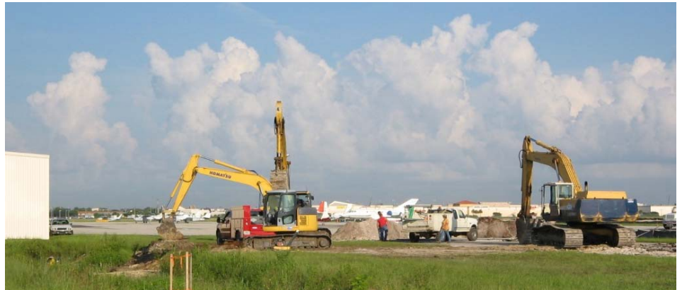
Taxilane Delta, closed to install underground pipes.
